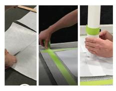
Pre-cut and dry fit fleece, prior to application. Tape all perimeters of penetration detail two inches beyond fleece terminations.
