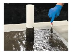
Once cured, apply a final coating of ALSAN Flashing at a rate of 2 gal/sq to the pipe and field, extending approximately one inch past the previous coat.
