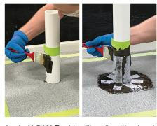
Apply ALSAN Flashing liberally with a brush at a rate of 2 gal/sq to the pipe, wrap the fleece around pipe or penetration and coat with an additional layer of ALSAN Flashing.
