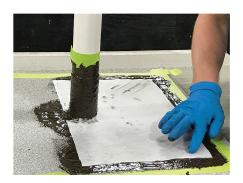
Apply ALSAN Flashing to the taped off field area at a rate of 2 gal/sq, lay fleece into the first coat and apply second coating of ALSAN Flashing. Remove the tape.
