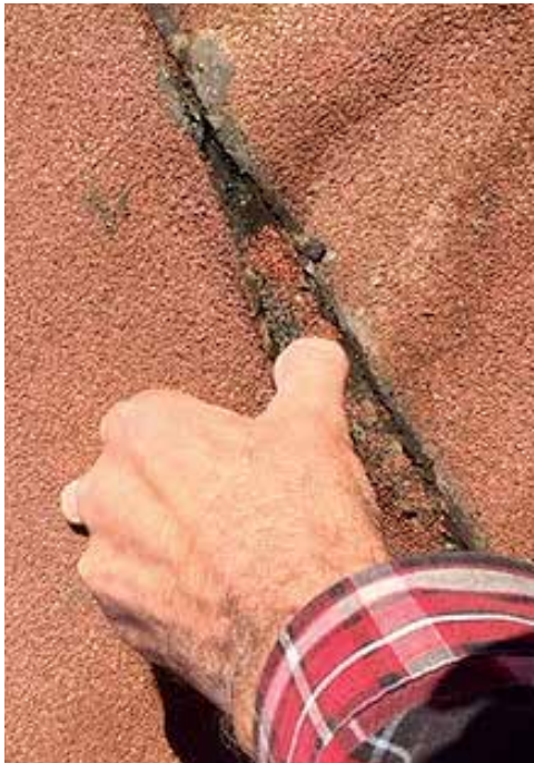
Membrane deterioration due to leak
