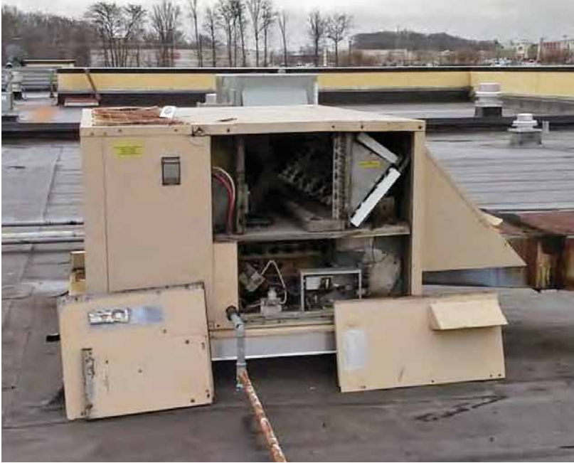
Doors need to be reattached to unit
