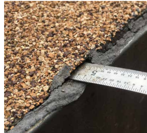
Gap in membrane at roof edge
