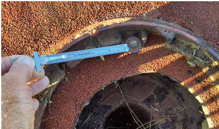
Loose drain clamping ring
