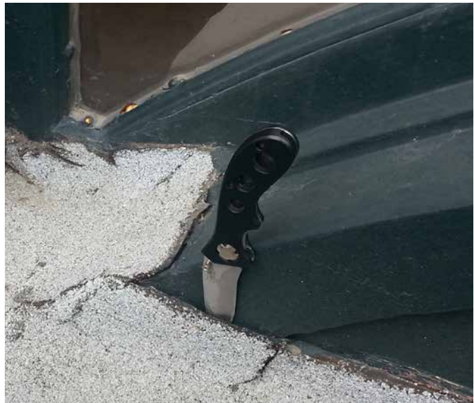
Membrane has pulled away from counter flashing
