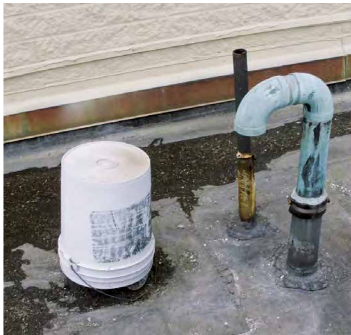
Not the correct way to repair leaking penetration
