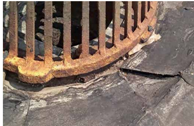
Open flashing lap around drain
