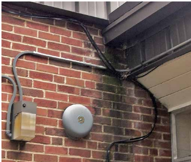
Signs of water drainage down outside wall
