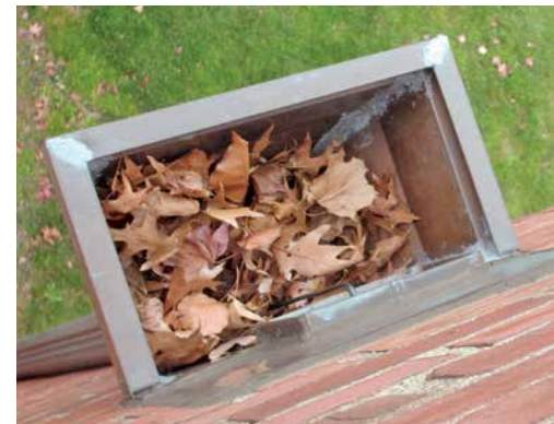
Check all gutters and downspouts
