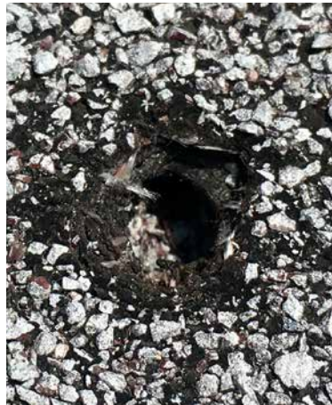
Puncture in roofing membrane
