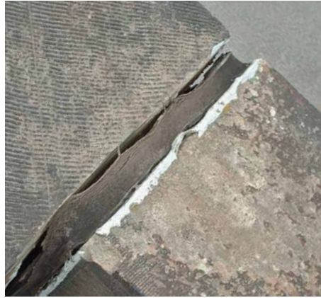
Detail of brick coping with cracked sealant
