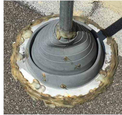
Pipe boot improperly installed
