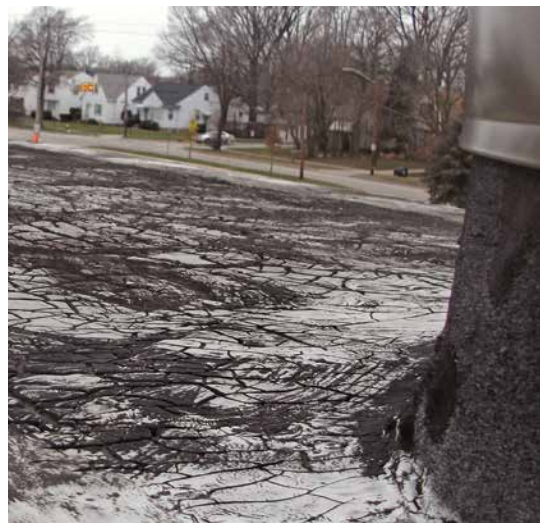
Cracked roof coating
