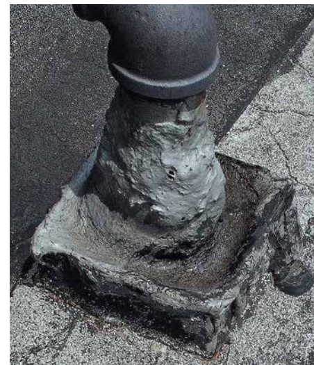
Pitch pan grout has pulled away from metal pan
