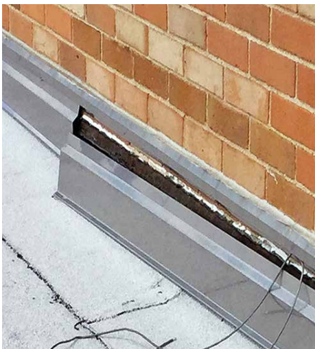
Termination bar that has pulled away from brick wall
