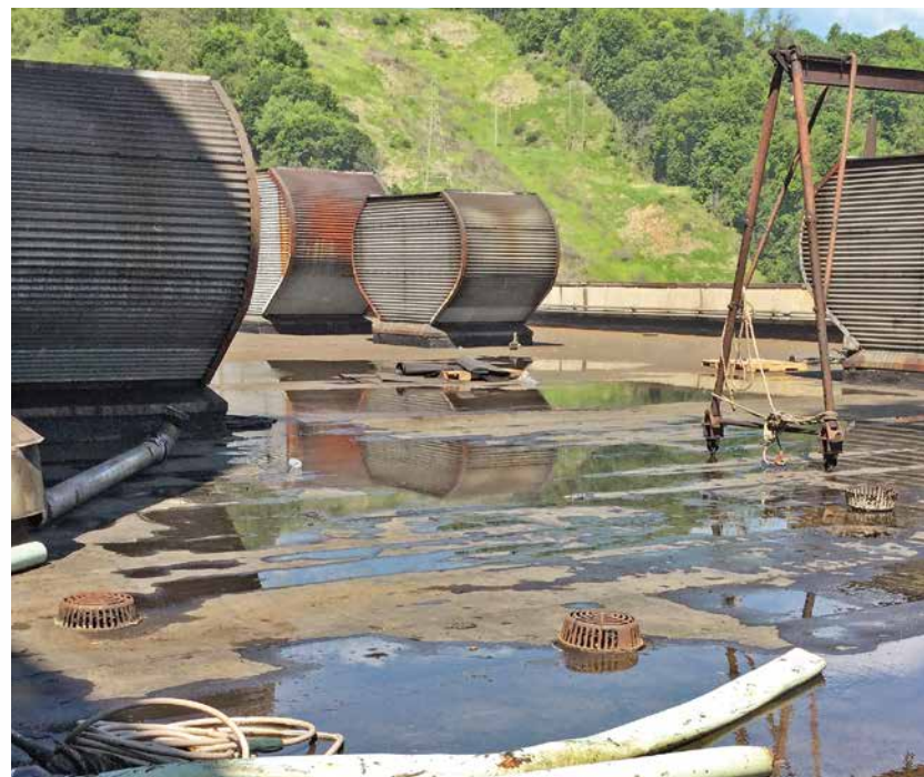
Standing water on roof surface
