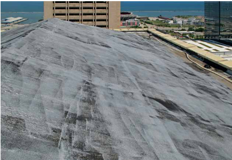
Worn roof coating
