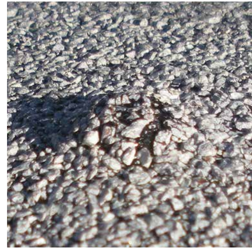
Fastener back out on granule roofing membrane
