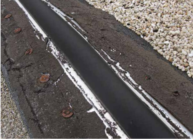
Exposed fasteners at expansion joint cover
