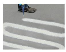
Hold the dispensing gun no further than 2 feet above the surface, spraying the adhesive in a ribbon pattern. Ribbons should be 2.5 inches wide and spaced 12 inches O.C. For complete application instructions and product specifications contact Technical Services.
